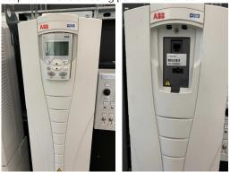
Step 1: Remove existing panel if installed.
