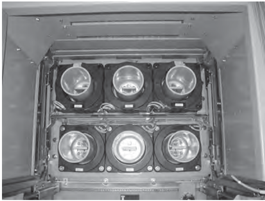
Typical CTs mounted in Power/Vac® breaker cell
