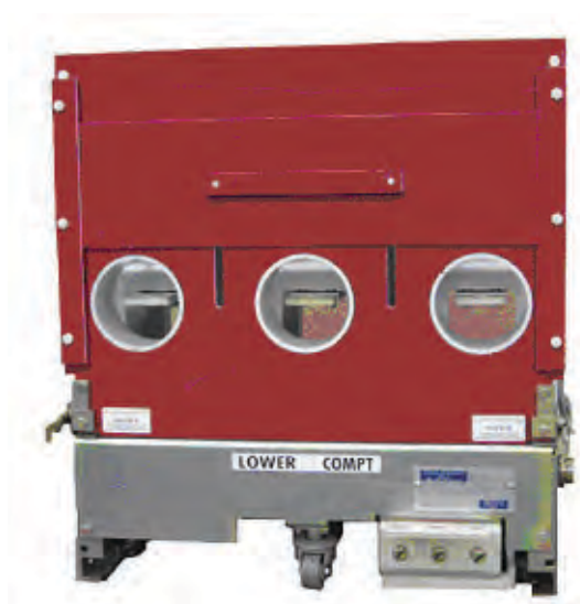
Figure 8-1 Standard Manual Ground & Test Device
