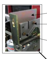
1- Connecting Bracket – Align 1<sup>st</sup> to existing holes in breaker frame.
