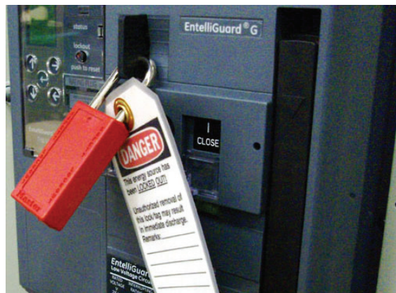
Figure 1.9: Breaker padlocked
