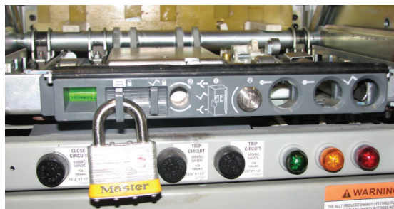
Figure 1.3: Primary disconnect shutters (locked in the closed position)
