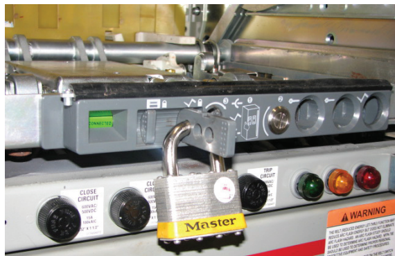
Figure 1.7: Rack padlocked
