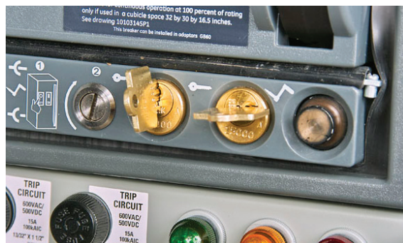
Figure 1.4: Kirk keys locking breakers (breaker in the CONNECT position)
