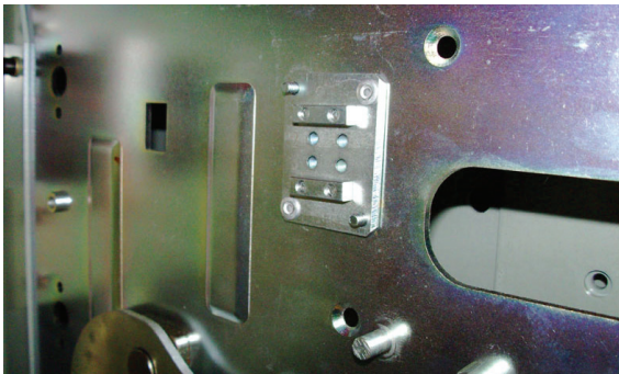
Figure 1.5: Breaker and cassette rejection (respectively)
