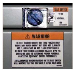
TEST Position: Momentary contact. Turns on the internal blue indicator, but does not engage RELT protection. The blue indicator is powered only through the TEST switch. It is not being powered by the trip unit output.
