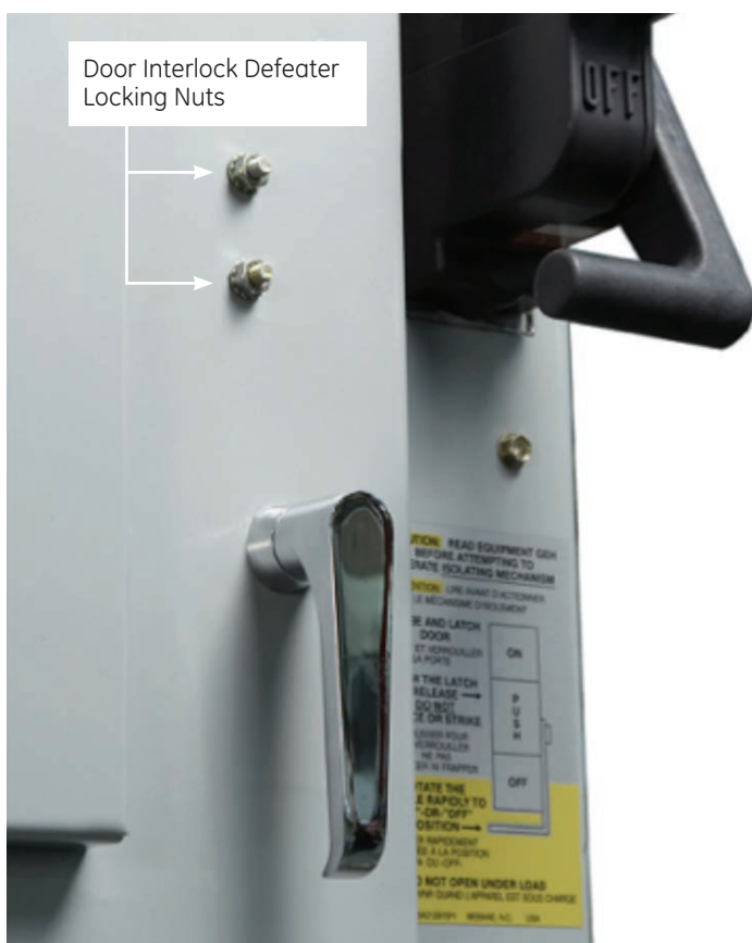
Figure 12. View showing door interlock defeater locking nuts.
