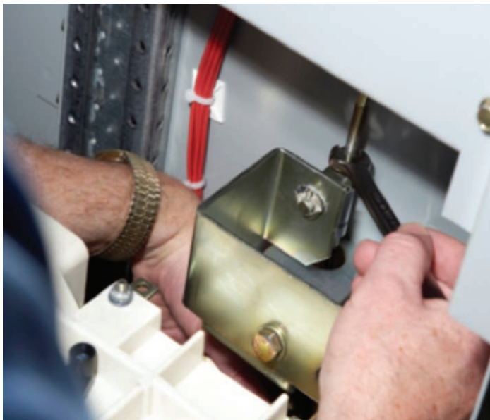
Figure 9. Adjusting connecting rod
