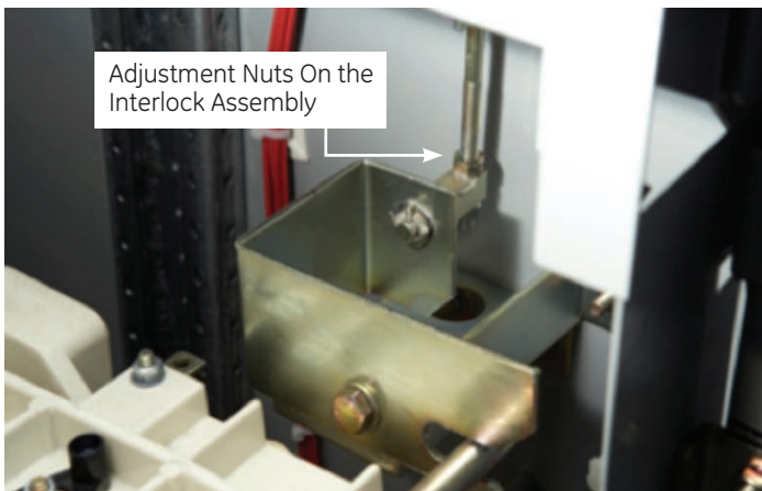
Figure 8. View of the contactor to isolation switch mechanical interlock at the vacuum contactor.
