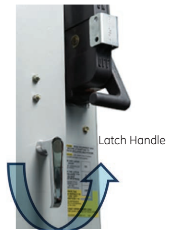
Figure 4. Rotating the medium voltage door latch handle.
