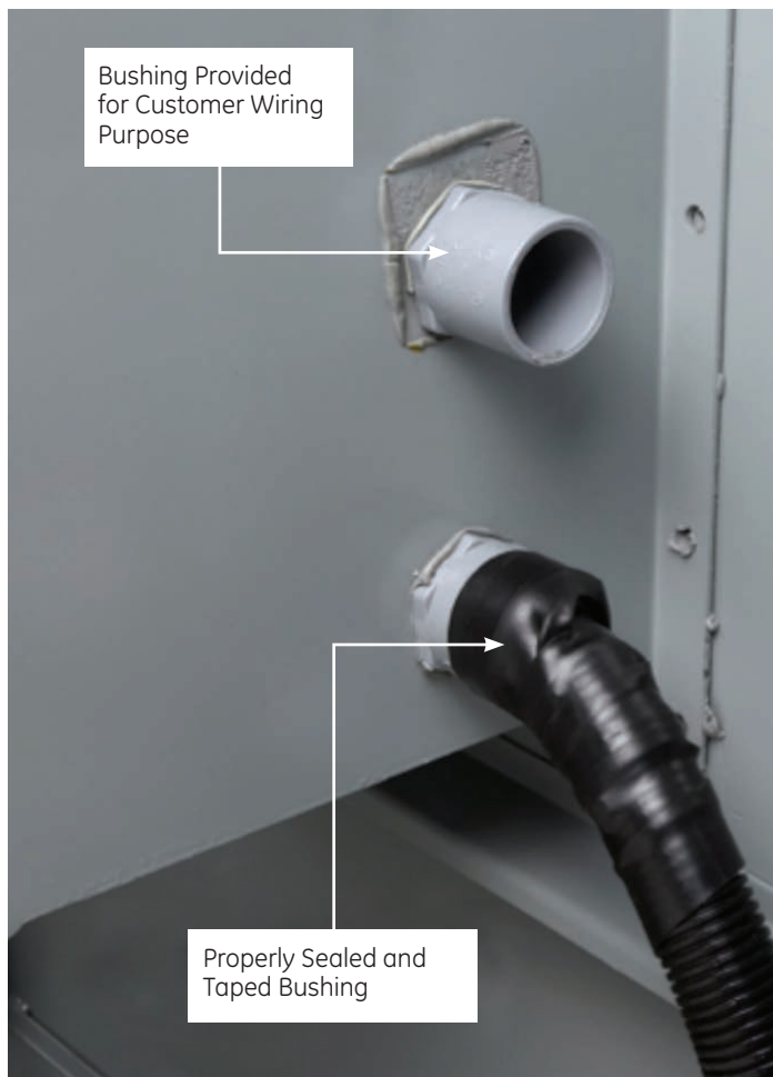
Figure 14. Low voltage box wiring.
