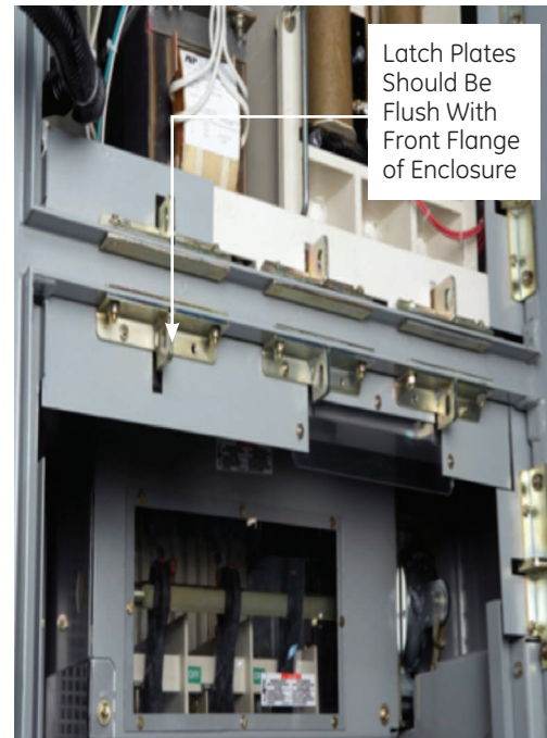
Figure 7. View of enclosure mounted latch plates.
