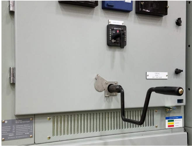
Figure 3-2: Circuit Breaker Manual Rack in/out
