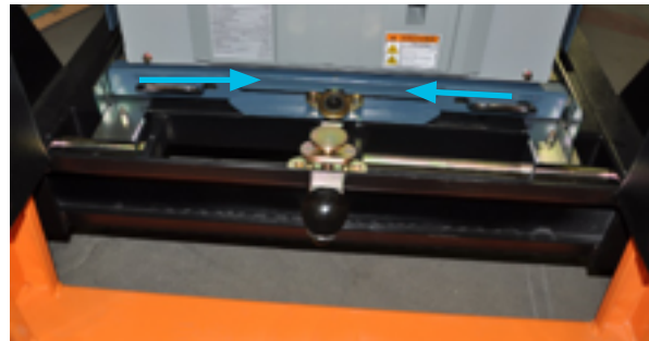
Figure 5-17. Unlock VCB from Lift Truck
