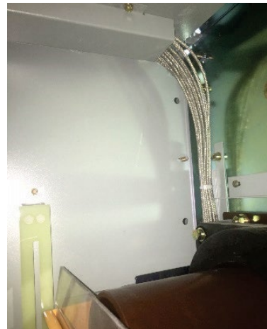
Figure 9-5: CT Wire Harness in Compartment
