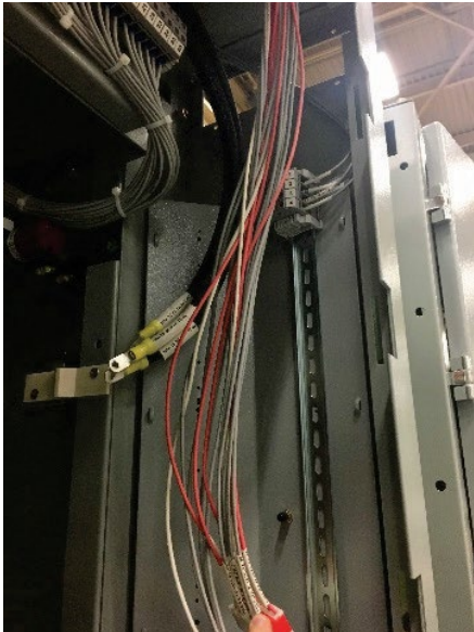
Figure 4-5: Position Wires for Clearance
