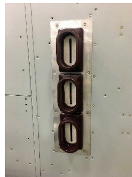
Figure 4-19: Side Bus Shrouds
