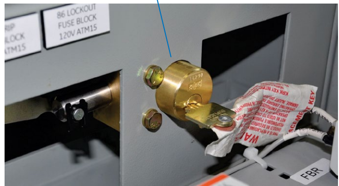
Figure 9-11: Kirk Lock Location in SecoGear
