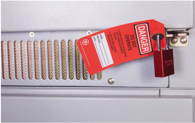
Figure 9-9: Compartment Door Padlock
