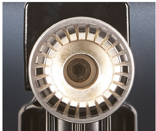
Figure 3-15: Disconnect Finger Cluster
