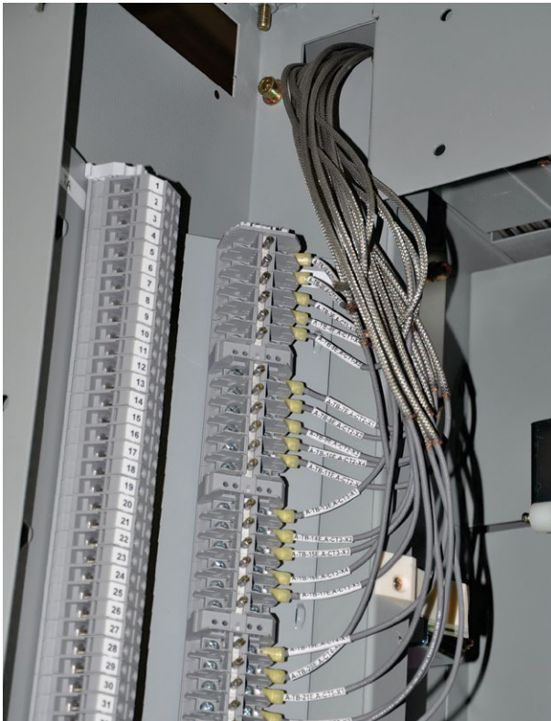
Figure 9-6: Shorting Terminal Blocks
