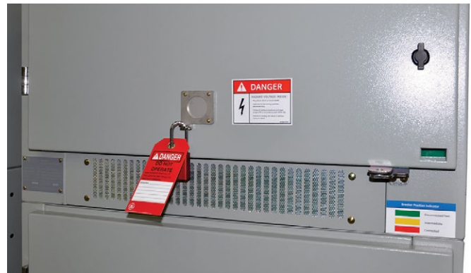
Figure 9-8: SecoGear Manual Racking Port Padlocked
