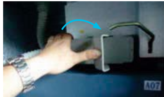
Figure 5-25. Insert Secondary Plug and Lock into Switchgear Compartment Socket
