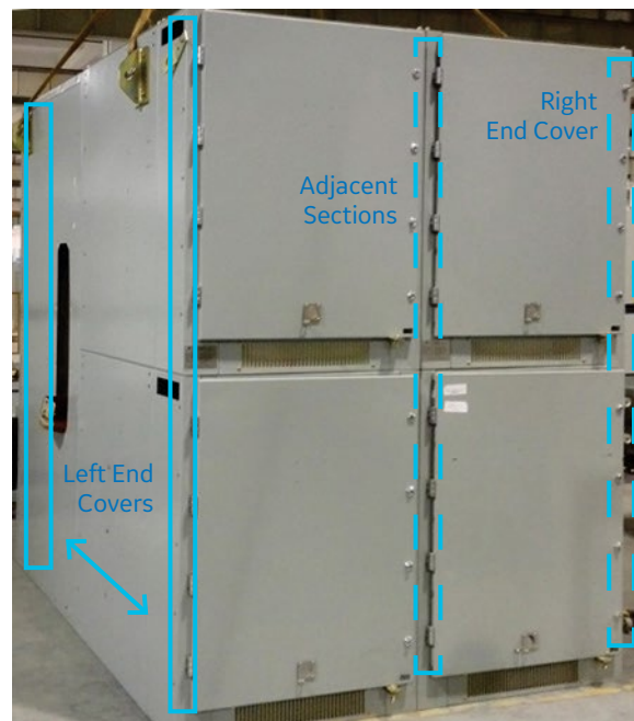
Figure 4-3: Lineup Shown Assembled
