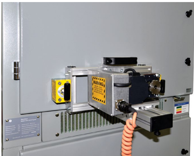
Figure 3-3: Circuit Breaker Automatic Rack in/out
