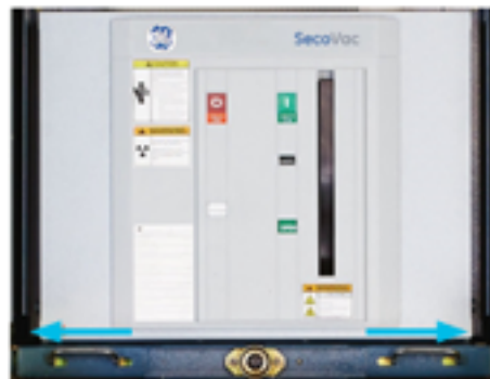
Figure 5-18. Lock VCB into Switchgear
