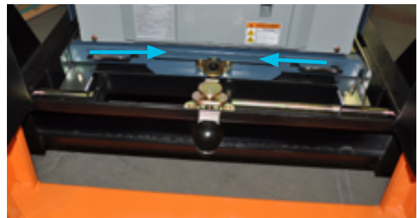
Figure 20. Unlock VCB from Lift Truck
