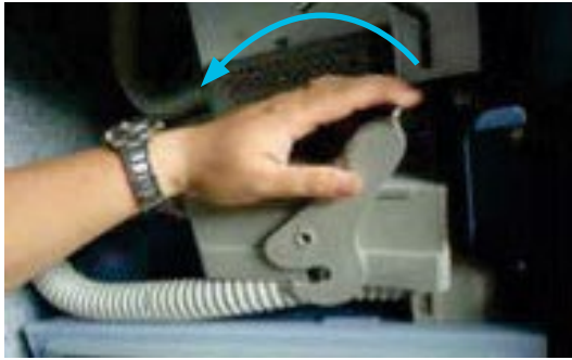
Figure 27. Release Secondary Plug from VCB
