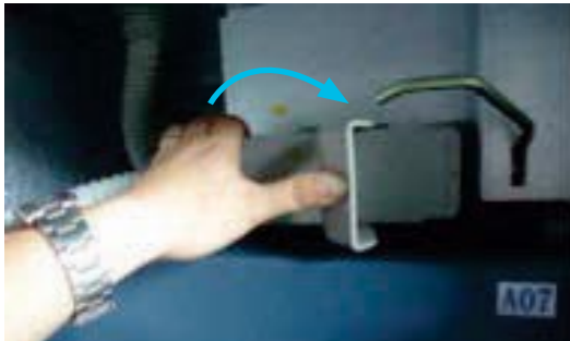
Figure 28. Insert Secondary Plug and Lock into Switchgear Compartment Socket
