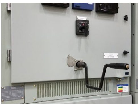
Figure 29. Racking Handle
