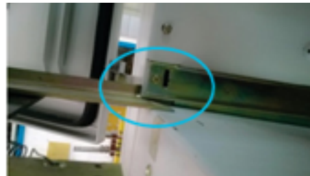
Figure 14. Lift Truck Arm (Left) Aligned with Switchgear Guide Slot (Right)
