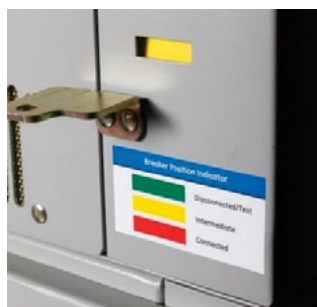
Figure 33. Intermediate Position (Yellow)
