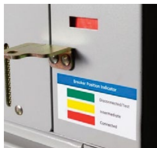
Figure 34. Connected Position (Red)
