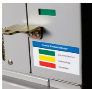
Figure 32. Disconnected/Test Position (Green)
