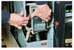
If the breaker is equipped with a MicroVersaTrip RMS 9 trip unit, the 36-pin trip unit connector must be removed and remounted on the adapter bracket provided. Slide the connector out of the mounting plate and install it on the adapter bracket, as shown in Figure 16-2.
