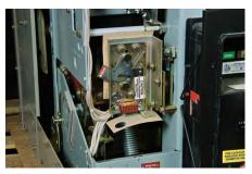
Align the connectors and rejection pin and connect the EntelliGuard TU to the circuit breaker, as shown in Figure 16-3.
