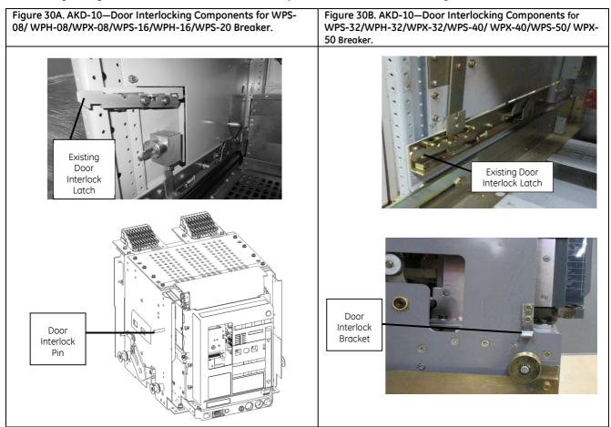
Details regarding installation of the door interlock system are shown below in Figure 30A and 30B.
