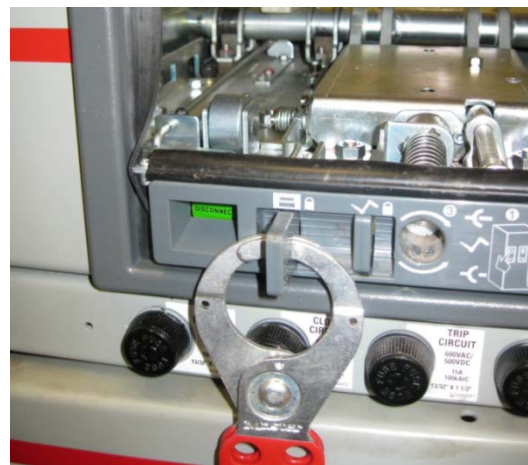
Figure 8.15 Circuit breaker shutter padlock device
