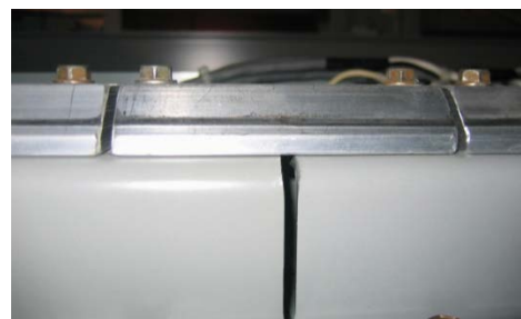
Figure 4.23 Front rail shipping splice installed
