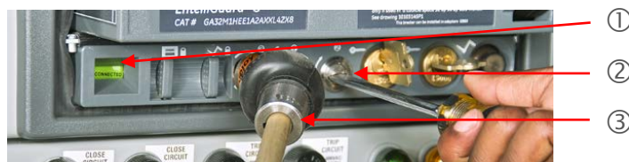
Figure 6.7 EntelliGuard racking handle
