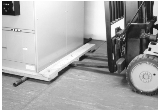
Figure 2.7 Method of rolling equipment
