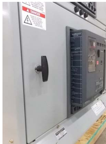
Figure 8.3 Circuit breaker in DISCONNECTED position
