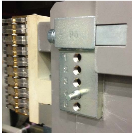
Figure 6.2 EntelliGuard circuit breaker rejection blocks
