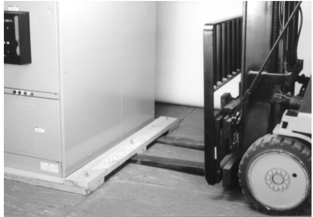
Figure 2.6 Placement of construction rollers
