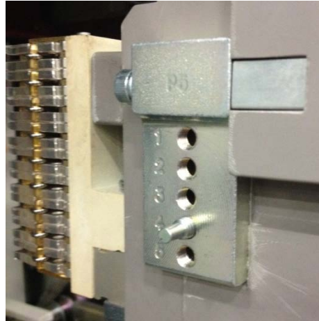
Figure B.2 EntelliGuard compartment rejection blocks
