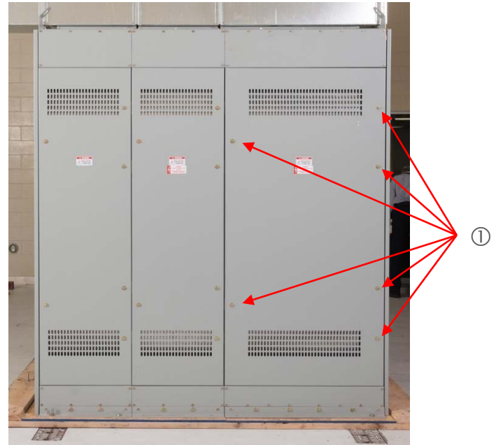
(1) Rear Access Door Closure Bolts (Typical)
