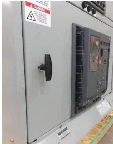
Figure 8.3 Circuit breaker in DISCONNECTED position
