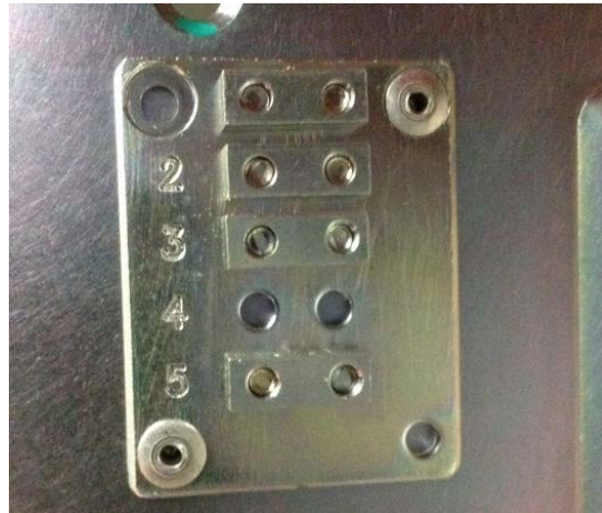
Figure B.2 EntelliGuard compartment rejection blocks
