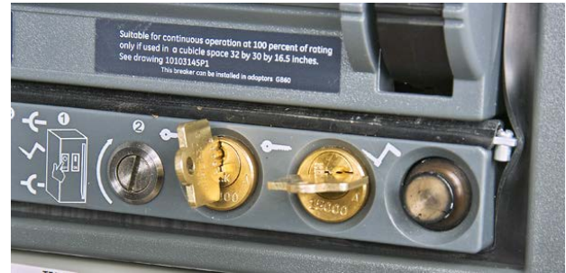
Figure 8.12 Circuit breaker key interlocks
