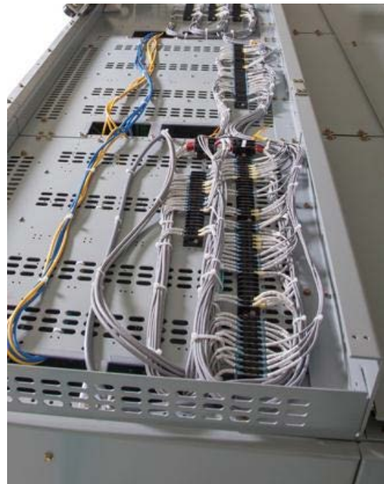
Figure 4.13 Interconnect control wiring
