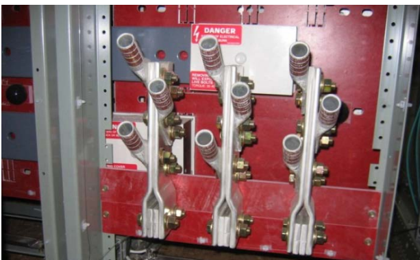
Figure 3.26 Cable termination provisions
