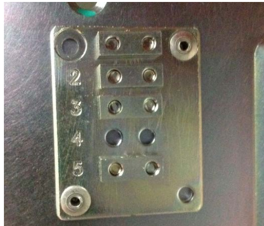
Figure 6.2 EntelliGuard circuit breaker rejection blocks
