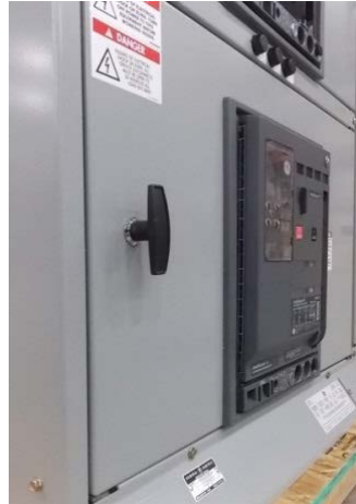
Figure 8.2 Circuit breaker in TEST position
