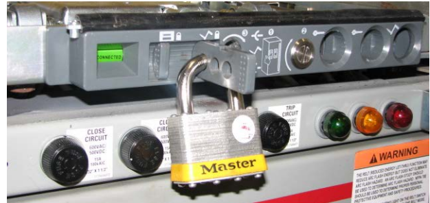
Figure 8.14 Circuit breaker draw-out rail padlock device
