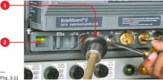
1. Racking handle 2. Breaker position indicator
