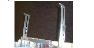
5. Using the hand grips on either side, pull the circuit breaker out of the cassette until it reaches a positive stop (rollers on the circuit breaker will stop against the extended rail projection as shown in Fig. 3.17).
