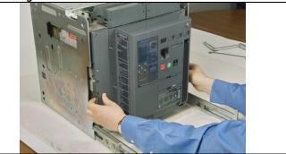
6. Attach the lifting bar to remove the circuit breaker.
