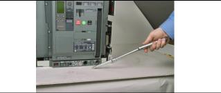
13. With a screwdriver, turn the racking handle shutter drive A clockwise (Fig. 3.14).
