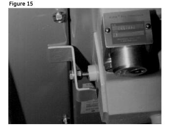
This interlock prevents the door of the enclosure from being opened when the switch is closed. When the switch is closed the door latch is, captured by the pivot of the operating handle, preventing the door from being opened. See Figure 15.
