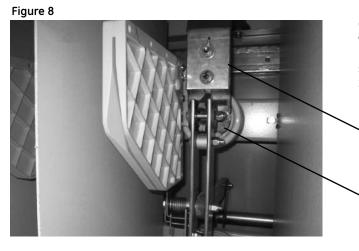
Check that the jaw casting contact surfaces align with the main blades. If necessary to adjust, loosen the jaw casting mounting bolts, tap on the spade terminal to align, then re-tighten the bolts. See Figure 8.
