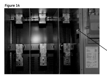
This interlock prevents inadvertent closure of switch if the enclosure door is open. When the door is closed, the push rod is depressed by the door to move the safety latch out of the blocking position. See Figure 14.
