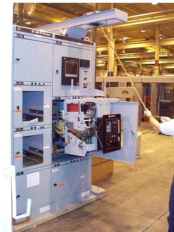
Fig. 5-5. Hoist breaker above rails
