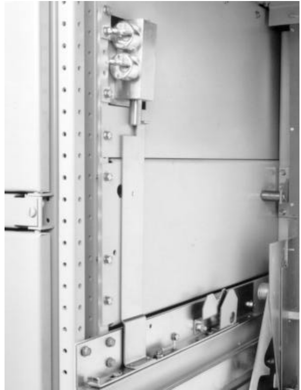
Fig. 7-5. View showing circuit breaker key interlock to provide protection against unauthorized operation
