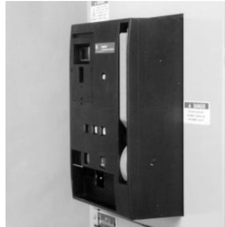
Fig. 7-1. EntelliGuard circuit breaker Shown in DISCONNECT position
