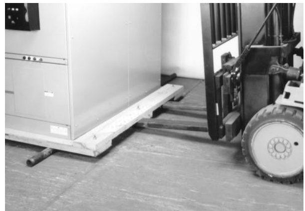
Fig. 2-5. Placement of rollers under shipping skid
