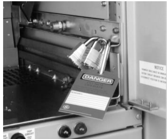
Fig. 7-8. Compartment padlock device (EG-08/16/20, EG-32/40/50 EG-32/40/50 FRE compartments)
