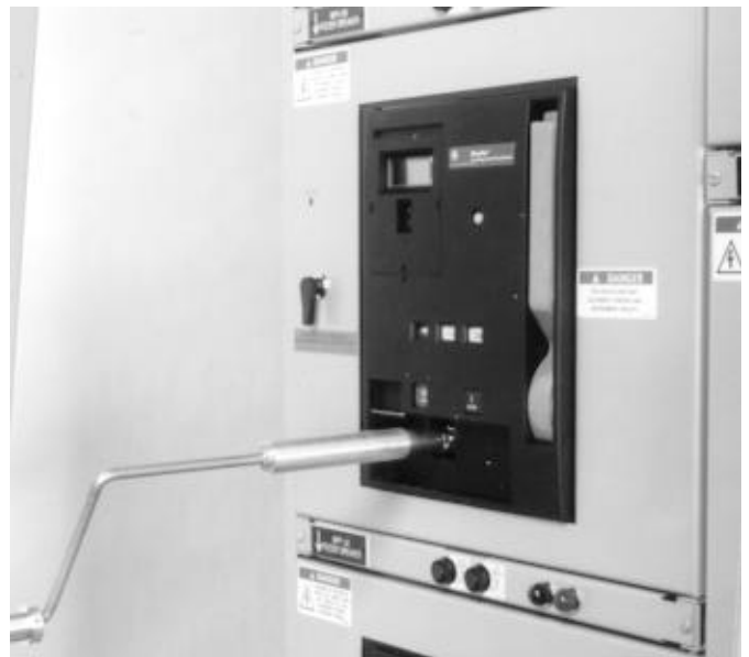
Fig. 5-9. Engage the racking screw with the racking handle
