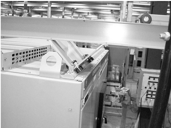
Fig. 4-22. Front rollers positioned on front track
