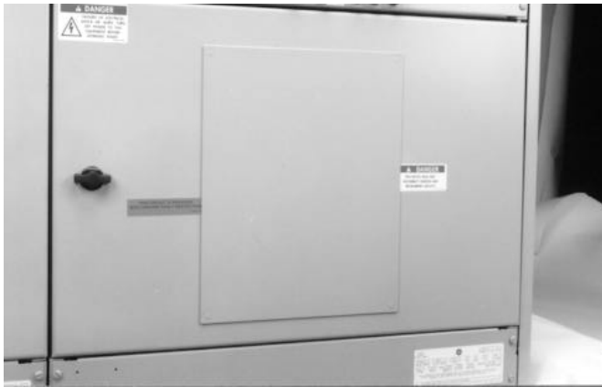
Fig. 7-4. Future-use breaker compartments
