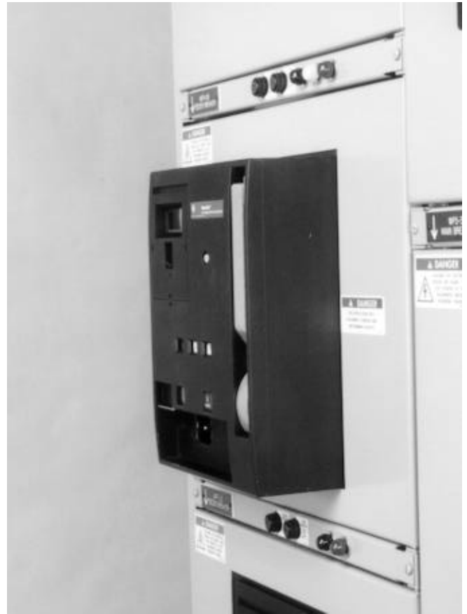
Fig. 5-8. Push the breaker in completely. Close the door.
