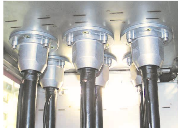
Connection of cables
