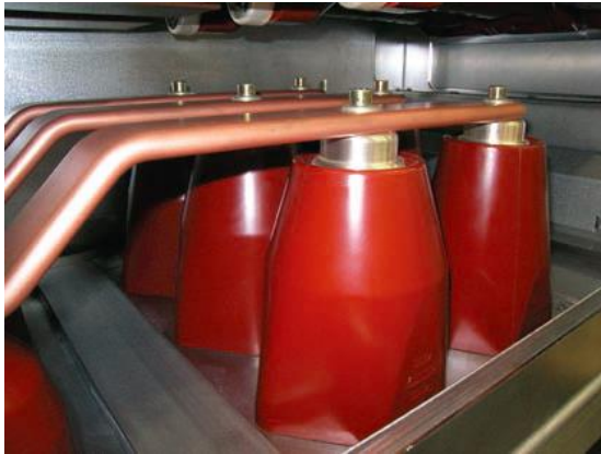
Inner cone termination
