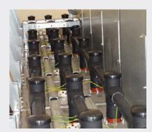
Busbar compartment with support for voltage transformers
