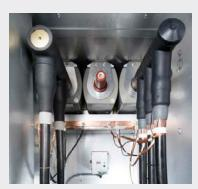
Cable compartment with current transformers
