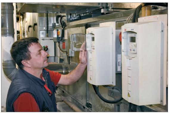
ABB standard drives for HVAC control the fans for the air conditioning system serving the two buildings that comprise the stadium's Quadrant expansion project.
