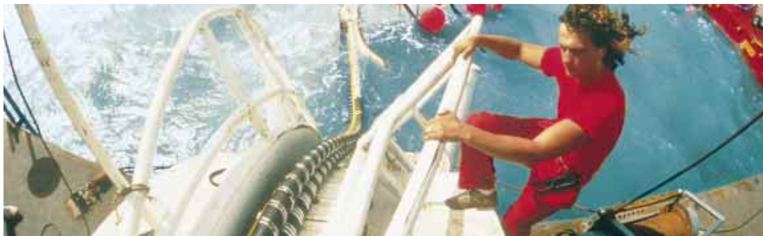
Laying of high-voltage submarine cables.
