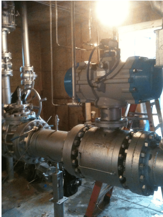
02 Distribution station control valve with ABB positioner
