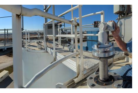
Laser transmitters are working reliably for powder silo inventory management
