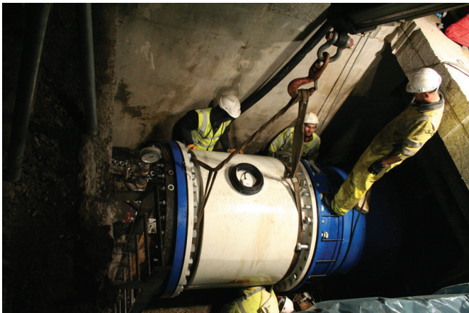
ABB's AquaMaster and WaterMaster flowmeters enable operators to choose between installation in a conventional chamber or direct burial.
