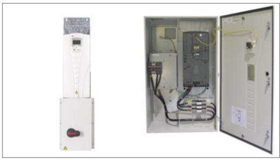
The ABB ACS550 Drive Package with Circuit Breaker (-PC) and Drive Package with Disconnect Switch and Fuses (-PD) offer users high-horsepower NEMA 12 solutions, and lower-horsepower solutions with disconnect options
