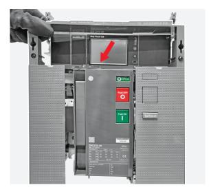
Manually remove the trip unit transparent cover.
