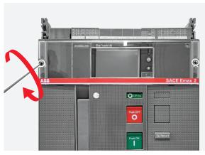
Manually remove the racking in and out lever located in the bottom part of the circuit breaker.
