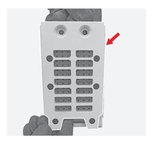
By means of the flat screwdriver unhook the 2 appendices fixing the arc quenching and the plate to the arching chamber main structure.
