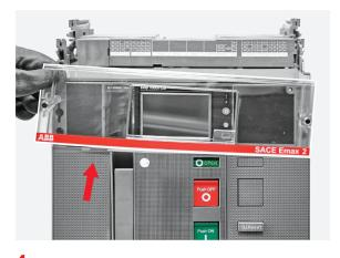
By means of the cross screwdriver unscrew the 4 screws fixing the front cover to the circuit breaker main structure.
