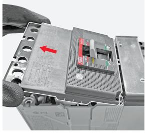
By means of the flat screwdriver push up the reset test rod and manually remove it.
