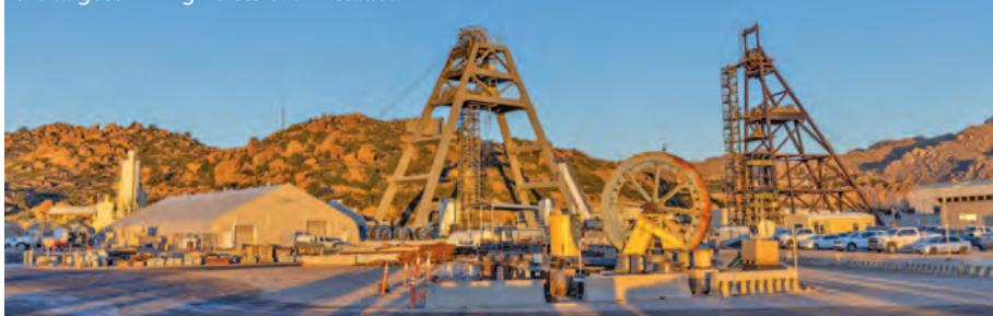
Resolution Copper's Shaft 10 will have one of the largest mining hoists ever installed
