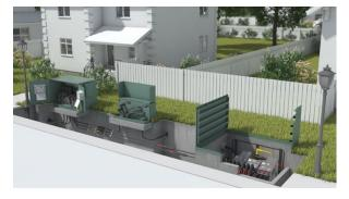
These designs are becoming increasingly problematic given safety concerns and the increasing threat of flooding, among other issues. Submersible apparatus and control systems represent one solution. Underground vaults should be designed to operate in floods, incorporating a water level monitor and a working pump and drainage system as well as a local battery system that maintains vault operations if source power is lost.
