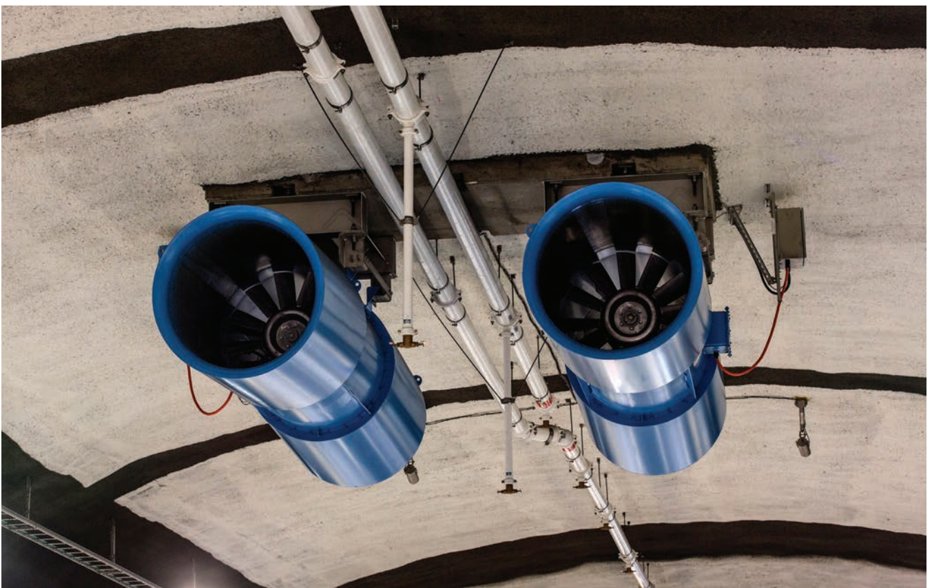
Above: A fan's smoke extraction motors must withstand high temperatures and continue to work reliably under extreme circumstances PHOTO: ABB
