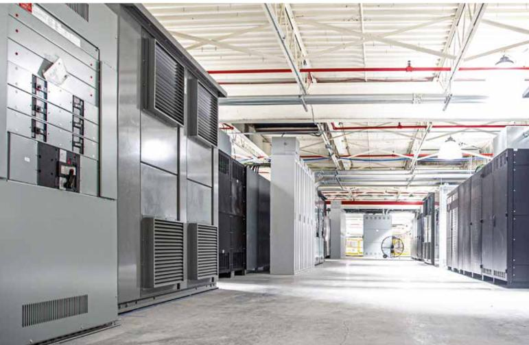
01 ABB and GIGA Data Centers developed an electrification solution of LV switchgear, dry-type transformers
