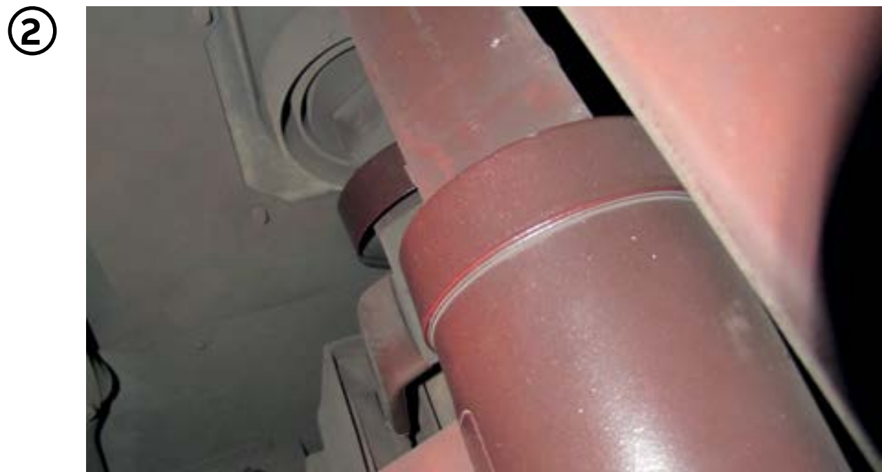
Ultra-fast earthing switch (UFES) 1) arc mitigation after 4 ms 2) arc mitigation after 90 ms
