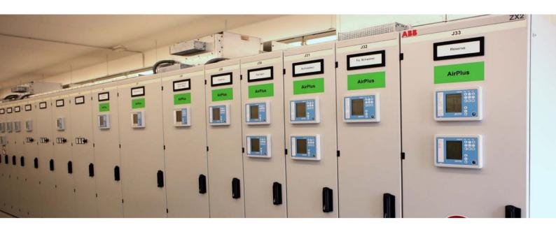
01 The dimensions of the ZX2 AirPlus panels are identical to conventional ZX2 panels and follow the same operation scheme. An ideal setup for the customer to compare both technologies side-by-side in real life operation.
