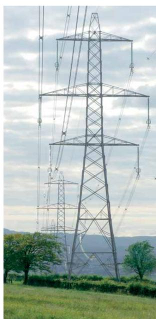
O1 Traditionally, expanding transmission line capacity was no trivial matter. However, the conversion of existing AC lines to DC allows extra capacity to be added without adding significant and costly new infrastructure or having to deal with the complexities of opening up new rights of way. (Photo: Anthony Byatt.)
