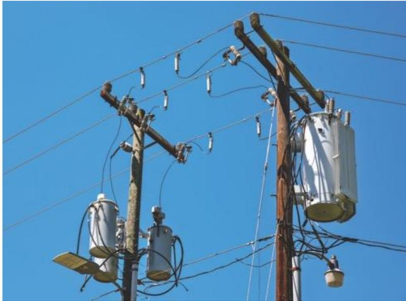
Backup fuse with pole-mounted transformer
