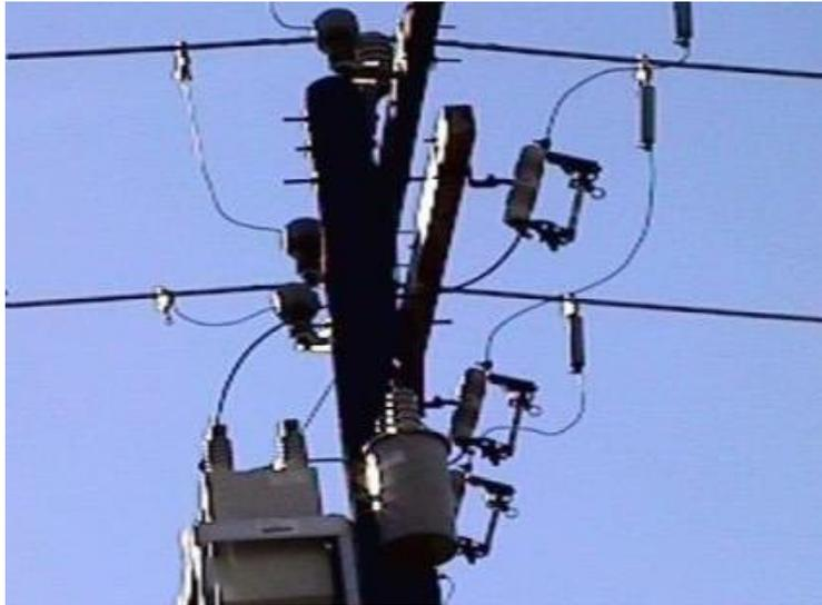
Two-fuse approach for protecting overhead capacitor bank
