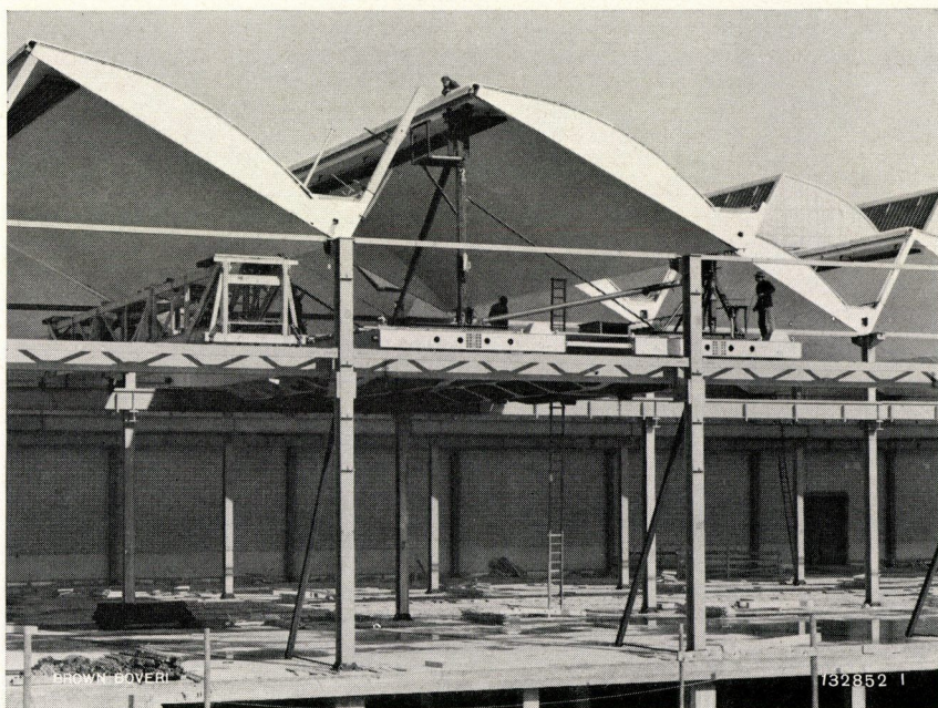
Fig. 6. — Moving a roof section into position
