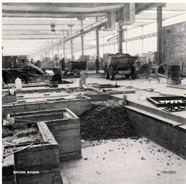
Fig. 5. - Foundations in the machine shop during construction
