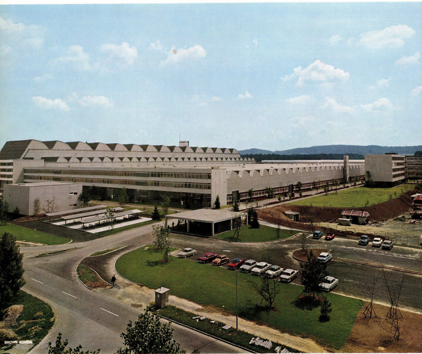
View from the north-west showing the factory extension and the new office blocks of the second building stage adjacent to the heavy engineering shop which has been in operation since 1960 and can be seen in the background.
