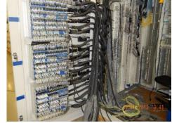
Figure 1 A data center low voltage compartment example showing conventional CT wiring for a bus differential
