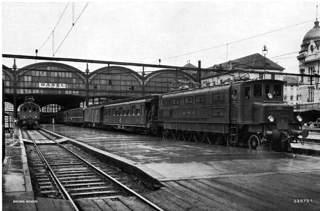
Swiss Federal Railways. Express passenger locomotive type 2 D0 1 with Brown Boveri individual axle drive.
