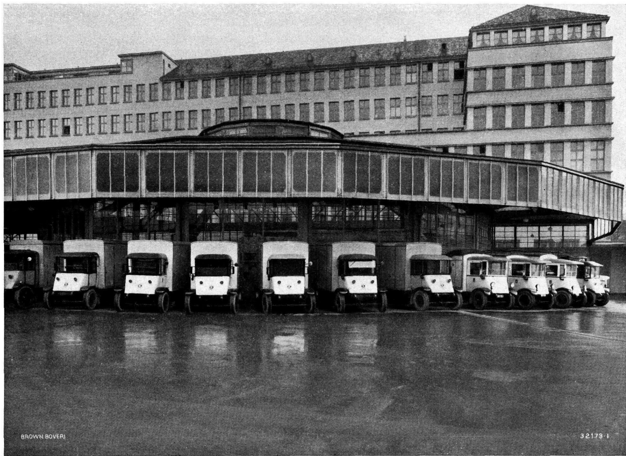
NEW GENERAL POST OFFICE (SIHLPOST) IN ZÜRICH. 62 charging stations for electric motor vans, fitted with the new Brown Boveri automatic charging equipment.
