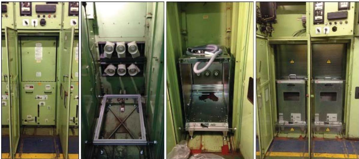
Fig. 5 Retrofill installation sequence
