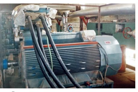
Switching from an old-fashioned steam turbine to a modern ABB rib cooled motor and drive package on its cane crusher helped Mirpurkhas Sugar Mills in Pakistan to reduce energy use by more than 40 percent.
