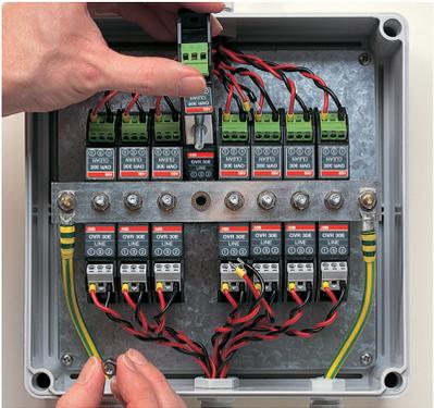
**Figure 2: Removing a SPD after installation**
