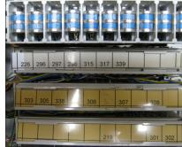
Clear the front face of the connection strip of all obstacles (eg label holders, magazines or gas tubes).
