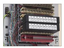
Figure 6 OVR protectors showing labels marked for line identification
