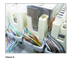
Connection of OVR KE10 to mounting frame, for earth connection.
