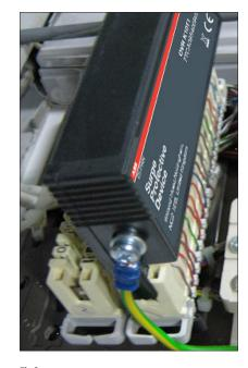
Fia 8: Earth connection to earth stud on OVR K10T1 or OVR K10T1/PTC.
