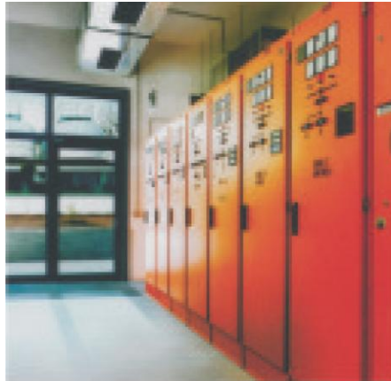
1984: First medium-voltage GIS with 3-phase encapsulation (ZV2)
