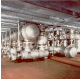
1967: World's first GIS switchgear High-voltage 170kV
