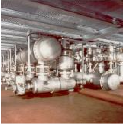
1967: World's first GIS switchgear
