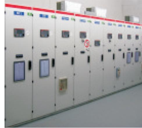
1994: First medium-voltage GIS without gas-works at site (ZX1)
