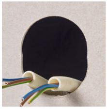
Pull out the flexible plastic conduits from the hole.
