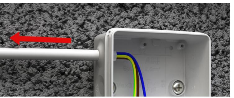
Pull cable back to seal entry. Box enclosure class IP65.
