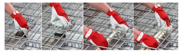
When attaching the boxes to plywood moulds, they can either be nailed or screwed.
