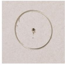
Do not drill the first hole completely.
