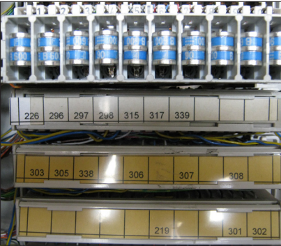
Figure 2: Clear the front face of the connection strip of all obstacles (eg label holders, magazines or gas tubes).
