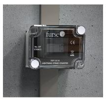
Figure 1: Furse ESP LSC-B secured to the down conductor of a building's lightning protection system.
