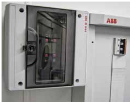
Figure 2: ESP 415 D1/LCD installed next to a power distribution panel in a suitable WBX D8 enclosure
