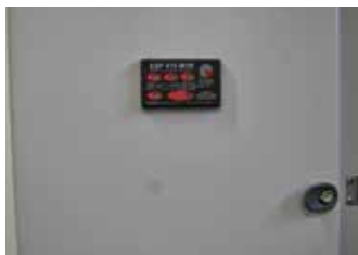
Figure 5: ESP 415 D1R/LCD remote display installed on the front of a power distribution panel.
