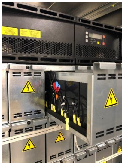
Fig. 7.4.1.6-1: Battery Drawer Reconnect
