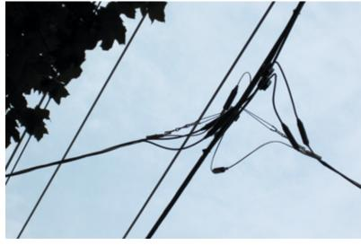
01 Pole installation: A typical Storm-Safe connection system attaches to a utility pole. Service connections and the attachment link are designed to release at the pole if a falling tree limb or some other heavy object strikes the lines. The de-energized lines are easy to reconnect.
