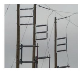
138 kV EXT current-limiting backup fuse in series with power expulsion fuse offers state-of-the-art protection. When properly coordinated, the Trans-Guard EXT current-limiting backup fuse always allows sufficient let-through current to cause the power expulsion fuse to melt and drop open, making it easy to visually pinpoint where the fault occurred.
