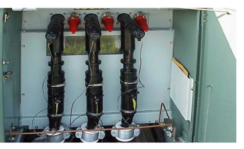
Industry: Electrical utility Challenge: Existing cable too short to reach bushing on new switchgear Product: Elastimold 600 amp replacement elbow
